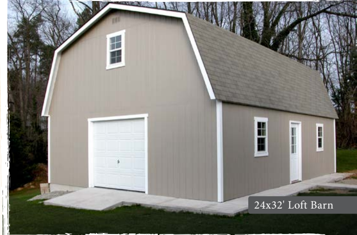
24x32' Loft Barn with metal roof and options
